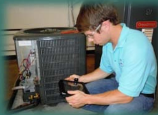
Heating, AC & Refrigeration
